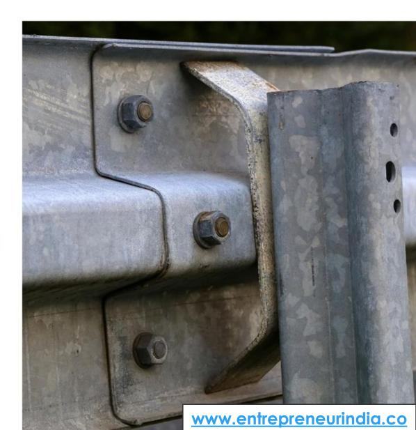
Metal beam crash barriers, also known as guardrails, are an important safety feature on highways, bridges and roads. They are used to protect drivers and pedestrians from potentially hazardous driving conditions. Metal beam crash barriers are made of metal beams or posts connected together with wire rope, providing a physical barrier that can absorb the impact of a collision or prevent vehicles from running off the road.
